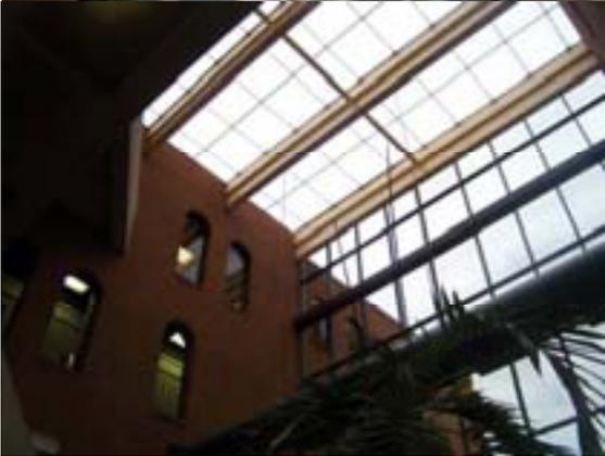
“We would recommend our 25mm triple-wall panel in clear, with the Lumira™ (previously known as Nanogel) aerogel filling. The clear panel because we want to let a significant amount of natural light into the room (or else, why to have a skylight). That panel will be UV coated on both sides, and most of the UV will be blocked by the polycarbonate. The remaining light will be diffused by the Lumira™ creating a softer light and equally distributing the amount of light in the room.”
