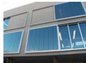
Gray polycarbonate panels. This created an operable shade-screen on the outside of the building envelope that could be operated by hand by the building occupants.
