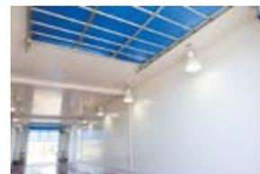
The tongue-and-groove interlocking system makes ease of both vertical and horizontal installations. A pre-punched nailing flange serves as a pilot hole; saving both time and dropped screws. The panel's half-inch thick wall design is lightweight and comes in standard and custom lengths. TRUSSCORE panels require no special training or tools to install and are safe to work with using normal construction practices. The waste material is also recyclable.
