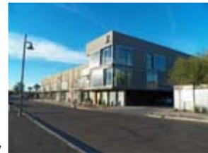
Completed back in 2004, the original building used CMU construction with fiberglass shade screens. In contrast, the new addition is a lighter, floating volume composed primarily of steel and EIFS. The expansion features an extruded aluminum frame suspended outside the façade.
