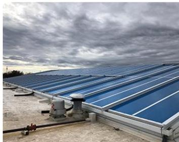
The motorized, retractable roof enclosure is approximately 140 feet by 70 feet, opens with the push of a button, and includes a rain sensor that closes it at the first sign of inclement weather.
