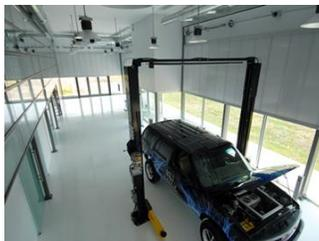
aerogel-filled LEXAN™ THERMOCLICK™ polycarbonate panels. These insulated motorized panels can be raised or lowered depending on the building's thermal insulation needs or to control the glare from direct sunlight.
